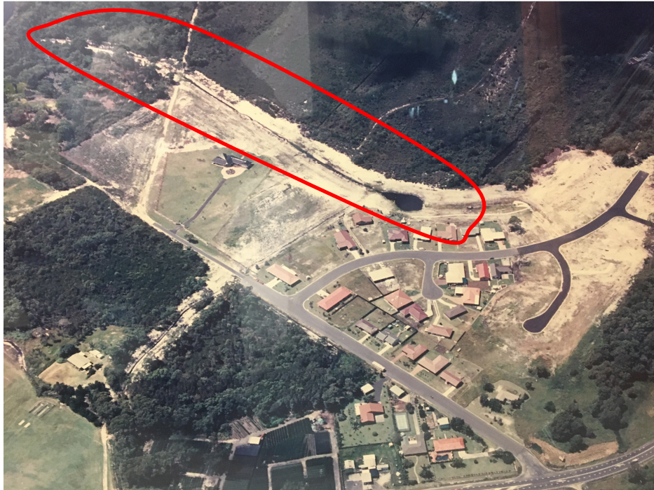
Plate 1 – Constructed Drainage Channel Circ 1992 (Refer RED markup)
