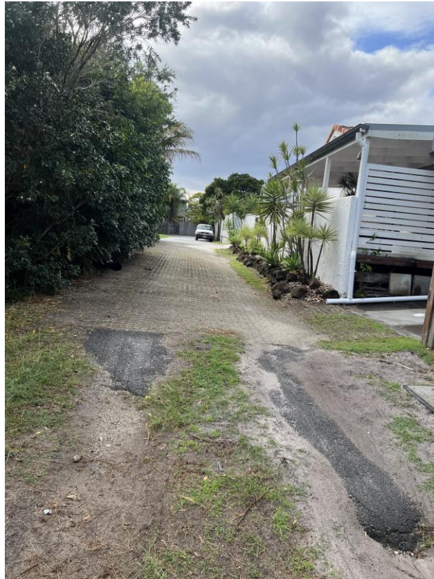
Figure 1: Similar development discharging stormwater to Somerset Lane directly
