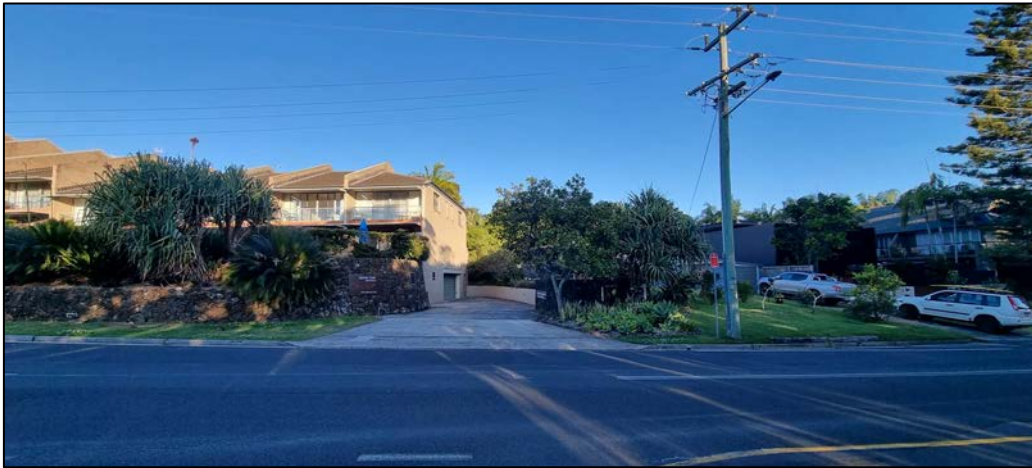
Photograph 1 – Residential flats and access driveway to the north of the development site within No. 130 Lighthouse Road).
