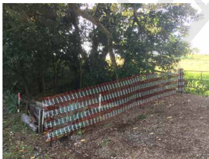
Figure 1. Example of high visibility temporary fencing.
