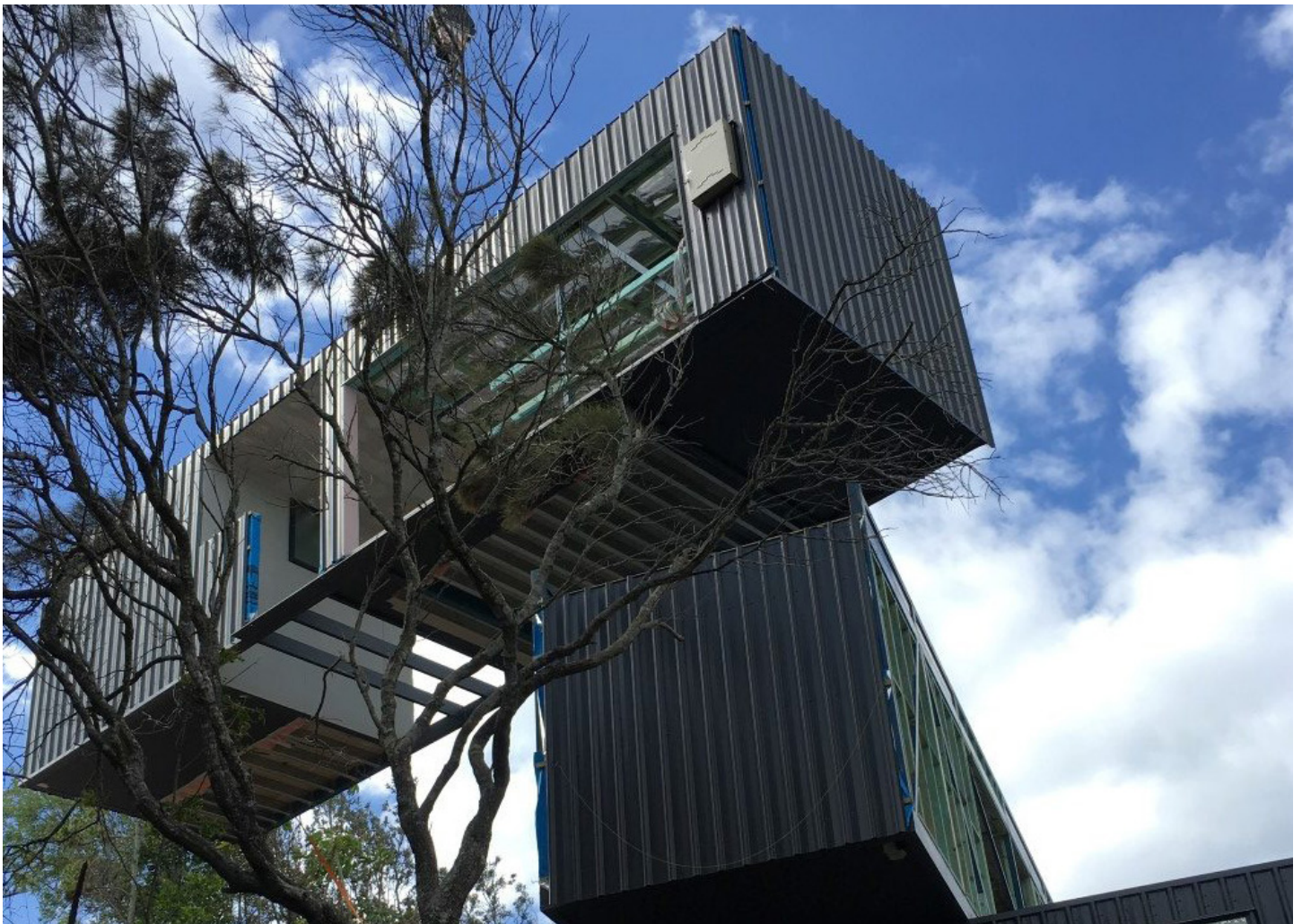
IMAGE: PREFABRICATION ALLOWS CONSTRUCTION TO OCCUR OFF-SITE IN CONTROLLED ENVIRONMENTS, MINIMISING WASTE AND DISRUPTION TO ON-SITE VEGETATION AND ECOSYSTEMS (SOURCE: BLOK MODULAR)
