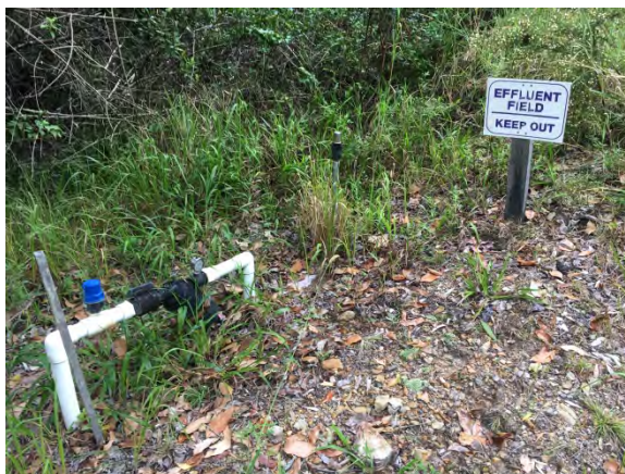
Photo 1 Irrigation infrastructure, PVC pipework manifolds and delivery lines, valves, pressure gauge, vacuum release valve and signage
