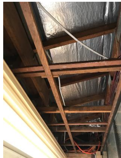
Plate3-4: Loading dock ceiling removed. No visible Ac debris remains on timbers or surface below
