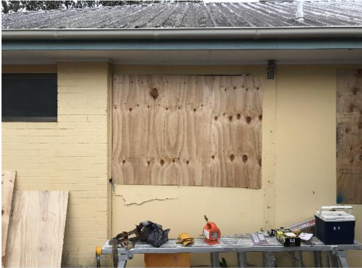
ID1: Both windows containing lead paint systems removed and disposed of.
