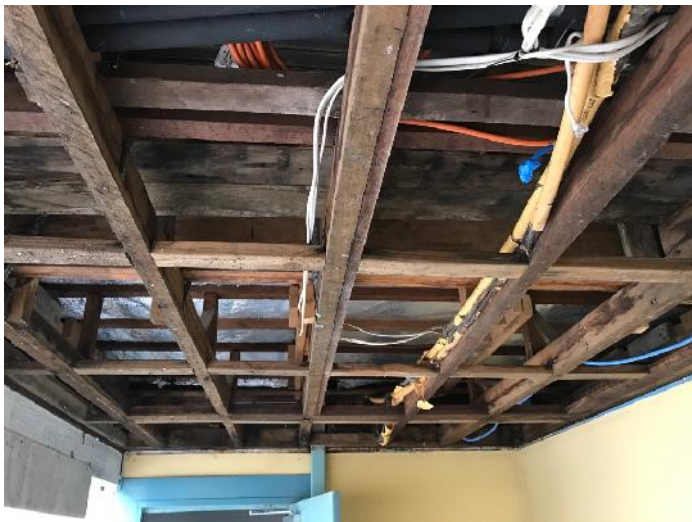
Plate3-4: Loading dock ceiling removed. No visible Ac debris remains on timbers or surface below
