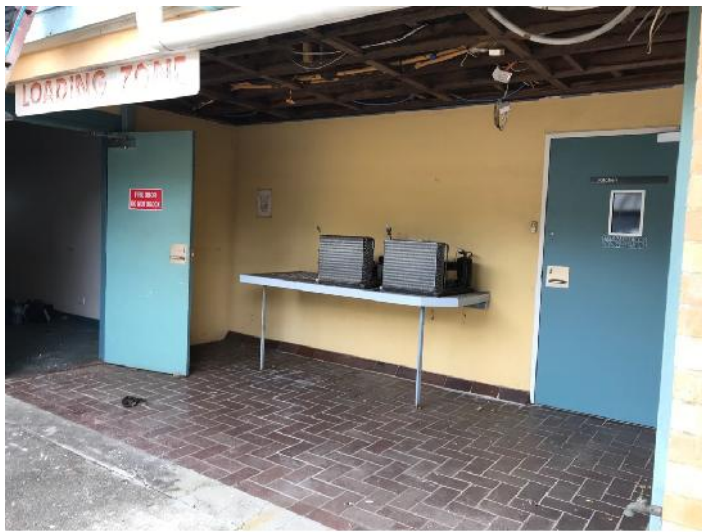
Plate1-2: Loading dock ceiling removed. No visible Ac debris remains
