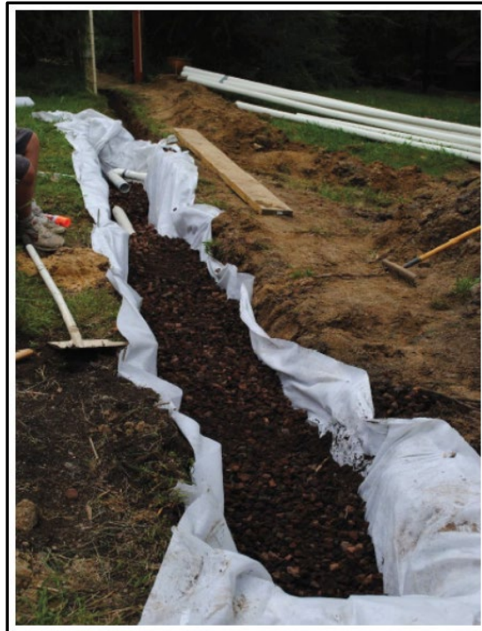
Figure 3: Underground Stormwater infiltration system.
