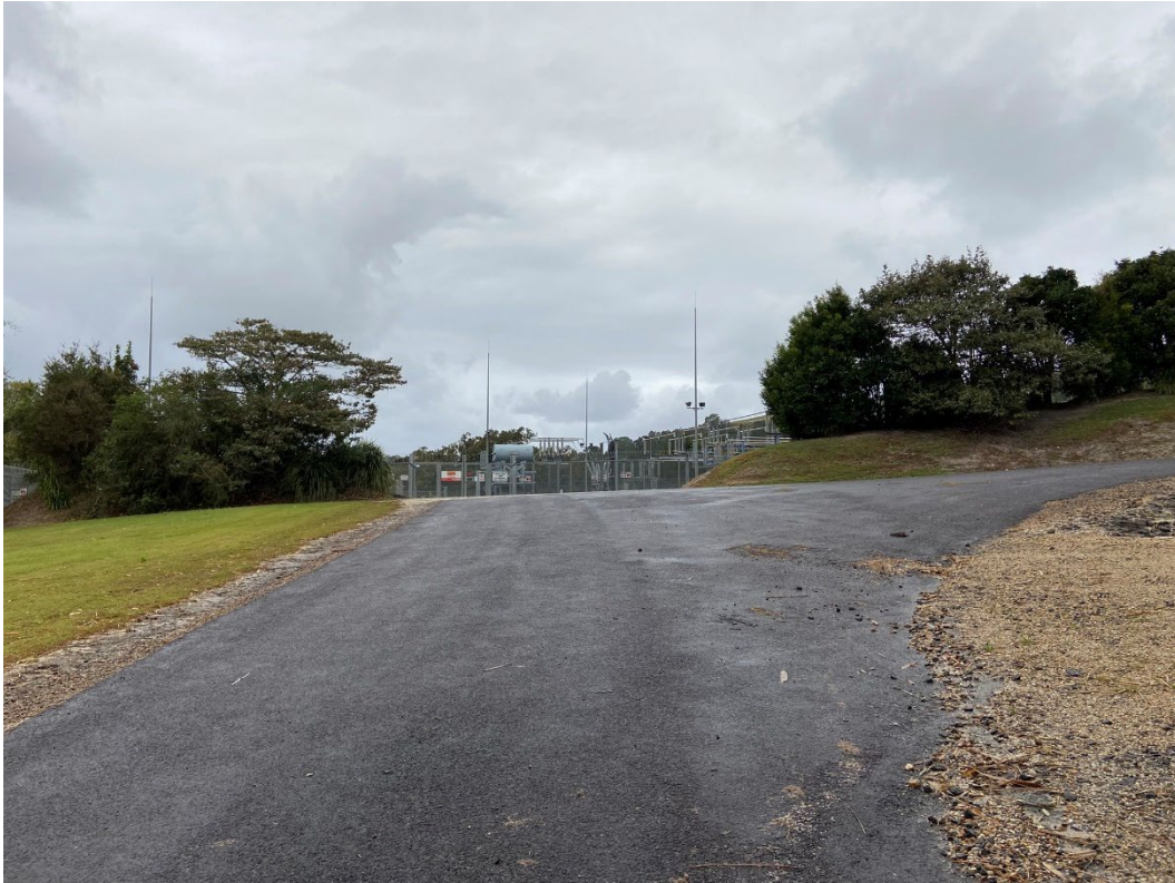
Photo C Essential Energy Substation located to the south east
