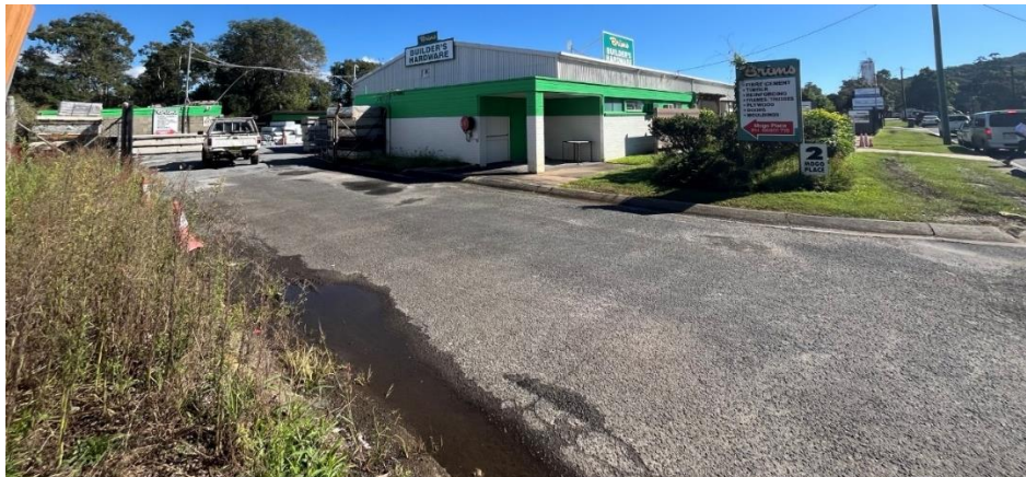
Figure 2 – Existing Northern Access to the Site
