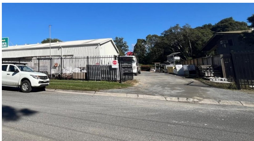
Figure 3 – Existing Northern Access to the Site
