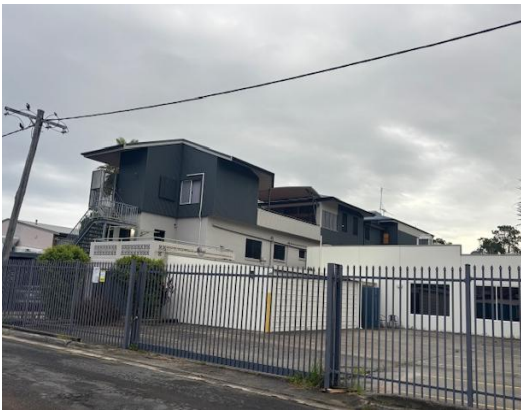
The rear car park and garages at 3 Fingal Street and existing three storey development at 1 Fingal Street adjacent to the site.
