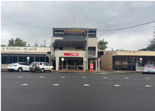
Existing three storey development located at 1 Fingal Street in centre of photo.
