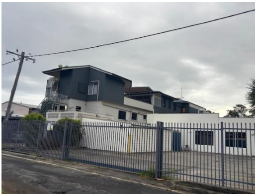
The rear car park and garages at 3 Fingal Street and existing three storey development at 1 Fingal Street.
