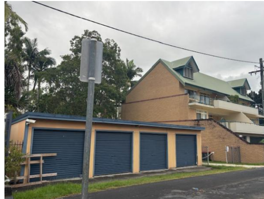
5 & 7 Fingal Street as viewed from Balun Lane.
