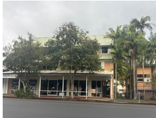
Development to the immediate west at 7 Fingal Street.
