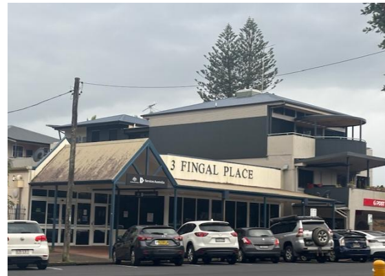
Existing development at 3 Fingal Street and 1 Fingal Street.
