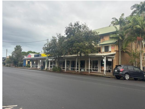
Existing three storey building to the immediate west, at 7 Fingal Street.
