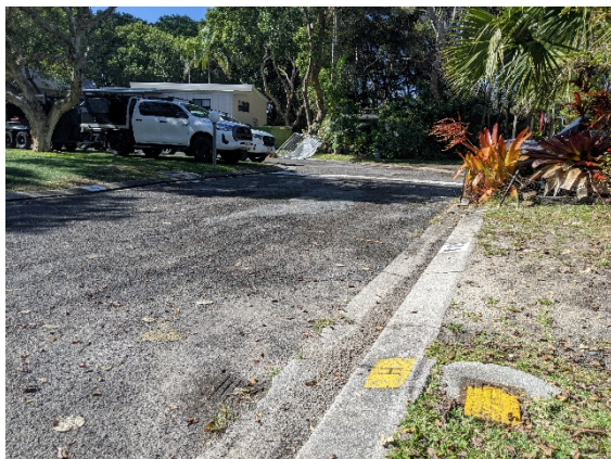
Plate 4.1 Hydrant on verge of internal access road
