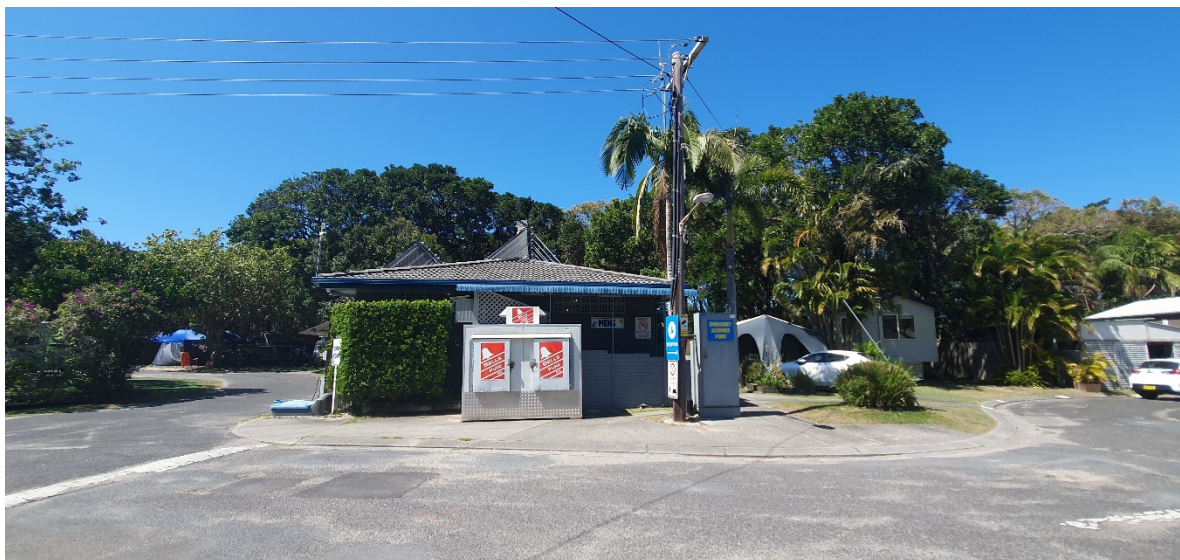
Plate 2.5 View east of existing amenities building
