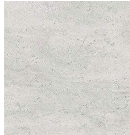
Off form concrete
