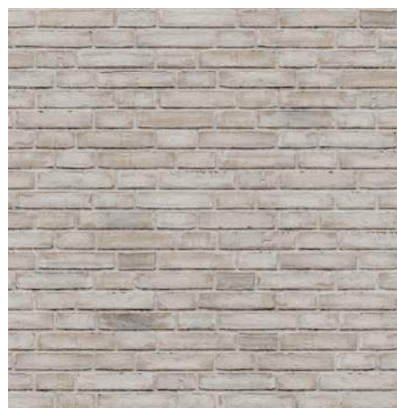
External Brick work
