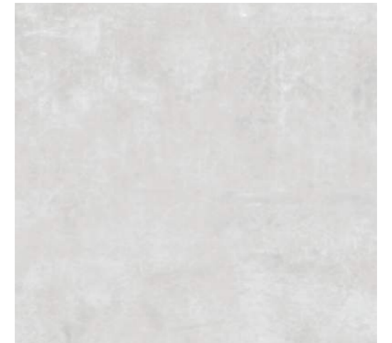
Off form concrete (CON01)
