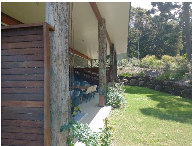
Photo 5 – outdoor living area along northern walls of dwelling. Retaining wall in background (see Note)
