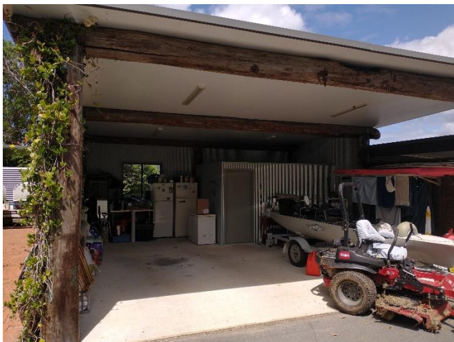
Photo 5 – Carport and laundry additions on northwest of dwelling (see Note)
