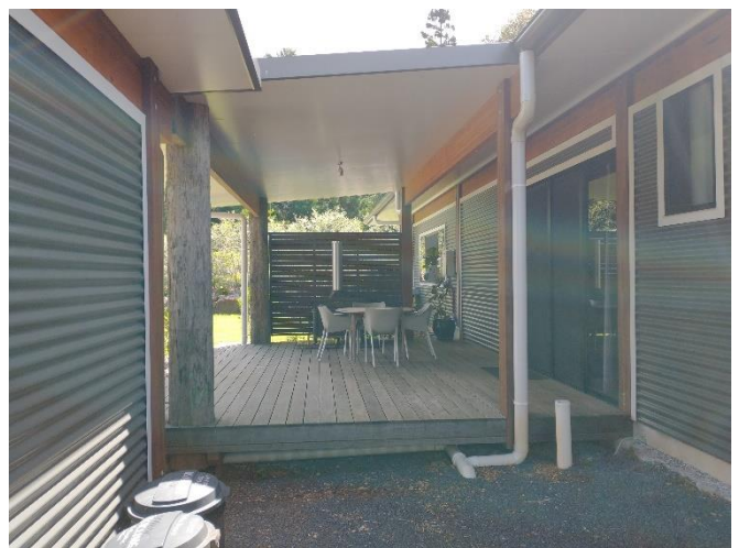
Photo 6 – Deck adjacent to carport and located on the southern façade of dwelling
