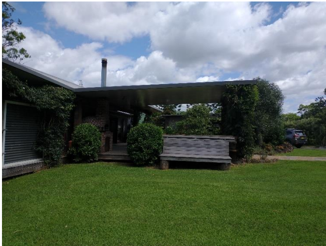
Photo 3 – ‘Outdoor living’ addition on north side / entry of dwelling
