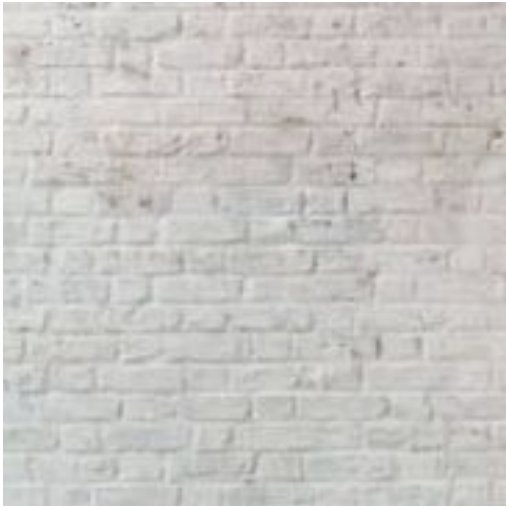
BRK.01: Cement bagged brickwork
