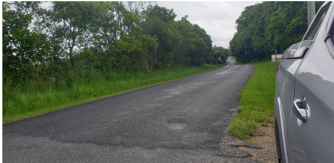
Existing access road to the property (Tyagarah Road looking west)
